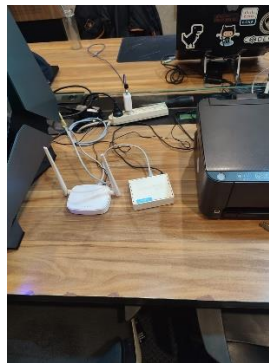
Figure 6. Mikrotik configuration with router
